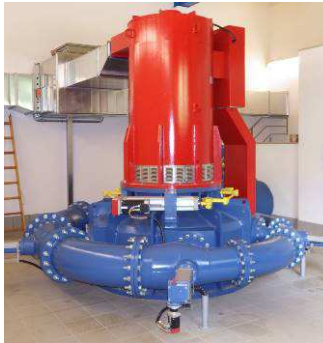
Pelton turbine/Generator
